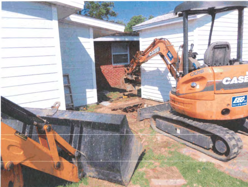
Picture 2: Excavation of UST 1167Jasmine.
